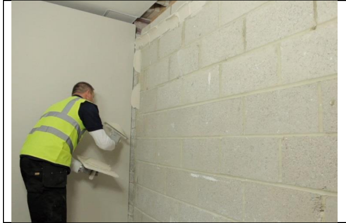
Figure 2 Direct bonding to wall
