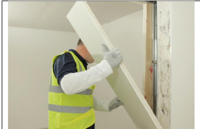
Figure 4 Window reveal installation
